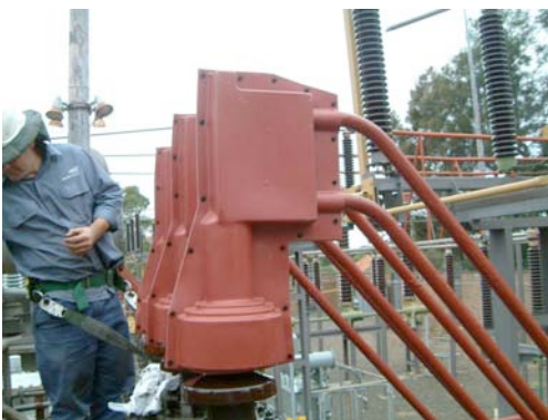
Figure 1 : Insulation Devices in a Sydney Substation
