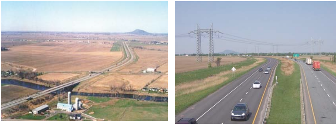
Figure 1. The line route was defined next to the highway for 37 km and it crosses it five times.
