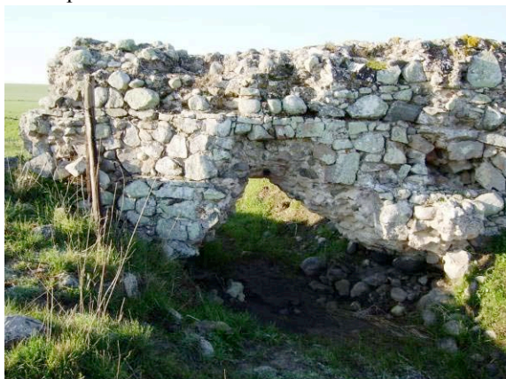
Figure 4 – This Roman Dam intersects a river bed which was supposed to be trimmed for a drainage network of an irrigation block but suffered only a mild intervention in order to preserve the classified monument.
