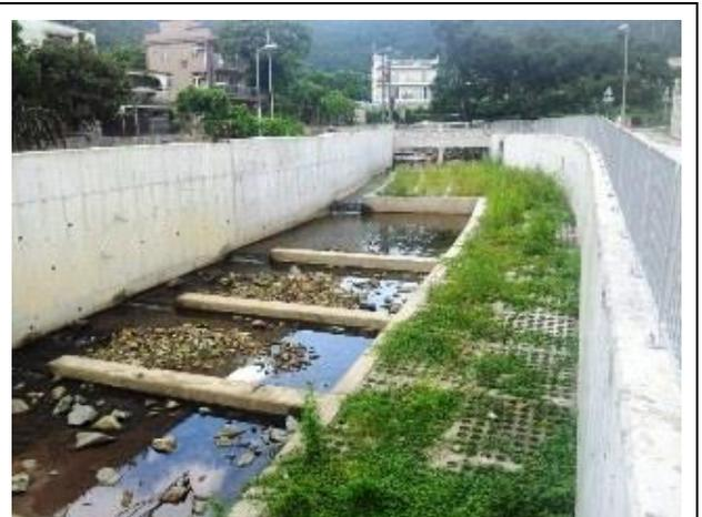
Photo 4. Kau Long Hang stream with ecology friendly design, after engineering works
