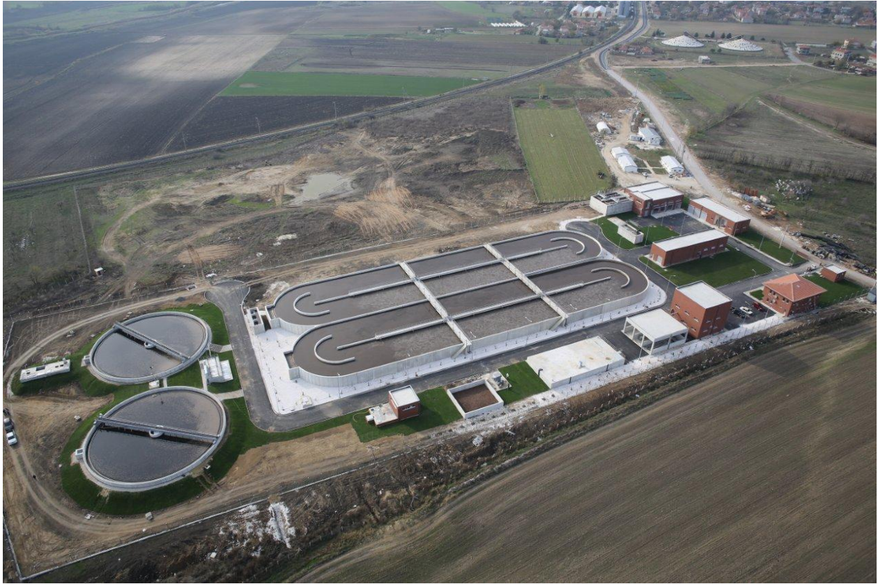
Figure 1: Photo from Lüleburgaz Wastewater Treatment Plant
