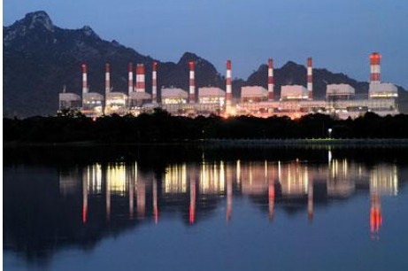
Source: Picture by EGAT via http://www.egat.co.th/
