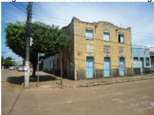
Figure 2 – Mansion before remodeling
