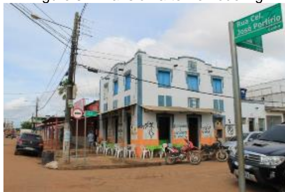
Figure 3 – Mansion after remodeling
