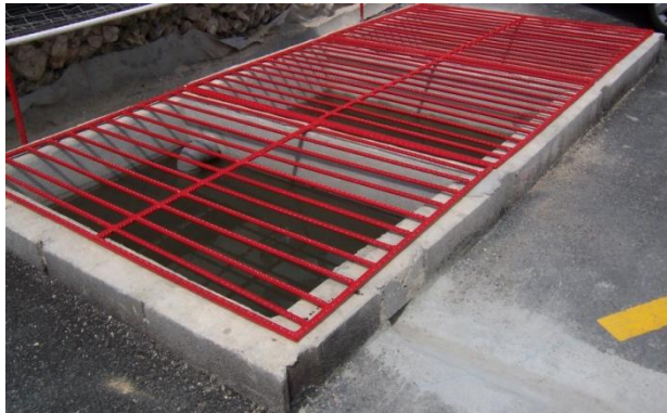
Treatment systems - sedimentation tanks
