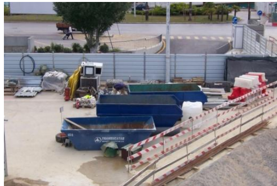
On-site sorting of construction and demolition waste
