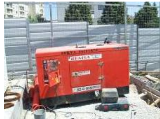
Site equipment far from noise-sensitive areas
