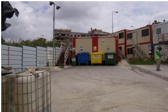
On-site sorting of construction and demolition waste
