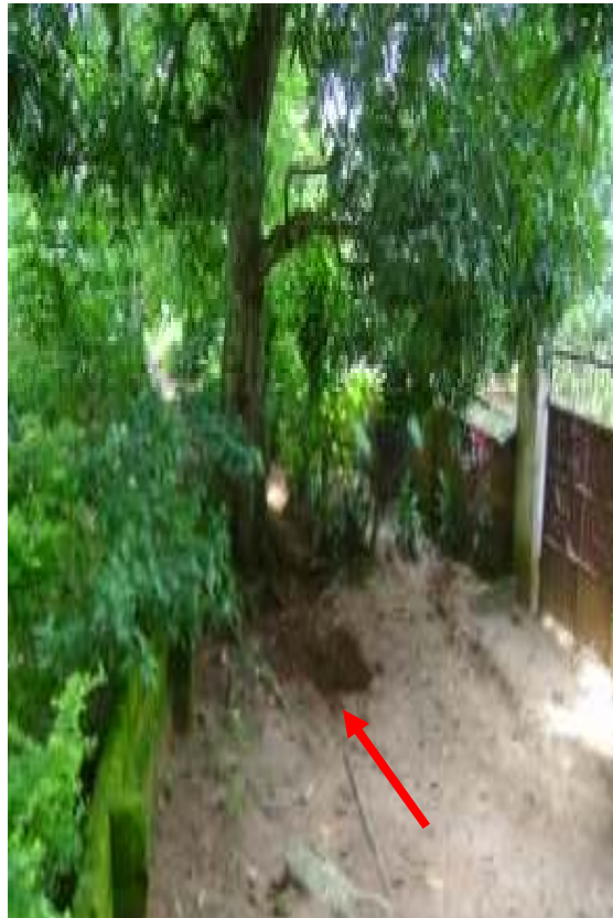
Shallow pits for reducing flood velocity
