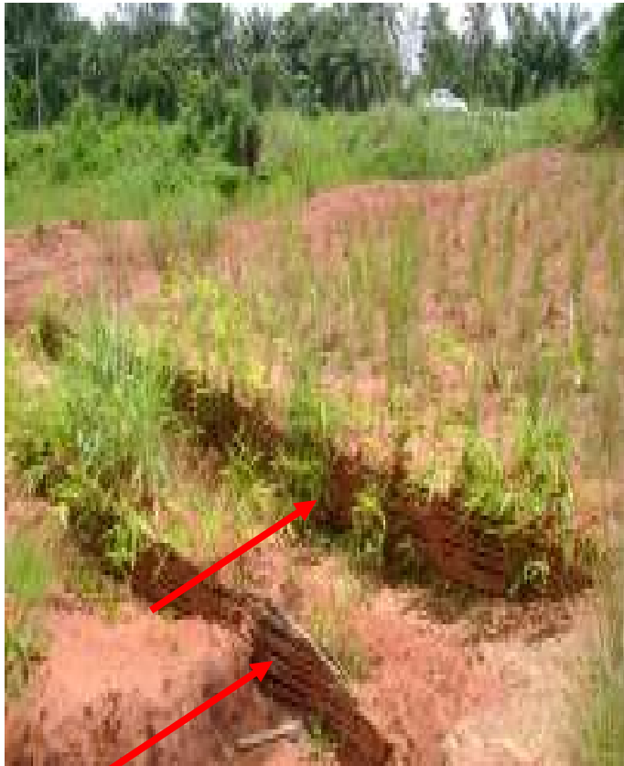
Use of locally made baskets and indigenous plant species for checking erosion and flood velocity
