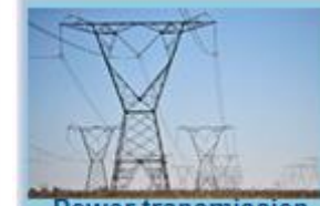
Power transmission lines
