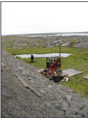
Drilling work, Puvirnitug
