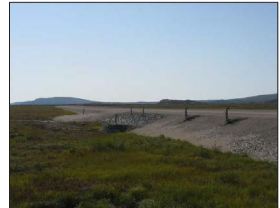
Test sections at Tasiujaq airport
