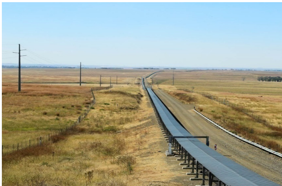
Figure 2: Typical example of an OLC on precast beams
