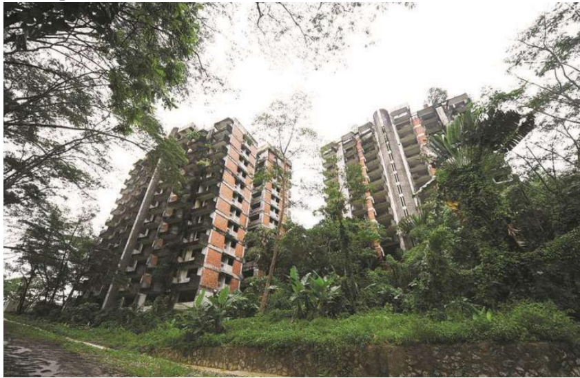
Figure 4 Remains of Block 2 and 3 of Highland Towers [24]
