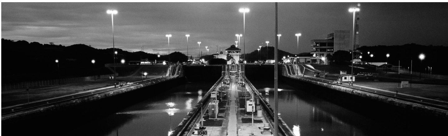
Miraflores Locks at dusk. Photo courtesy of ATP.
